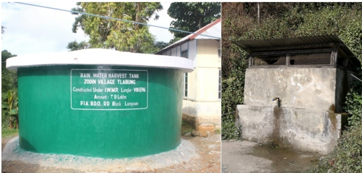
Figure 4: Rain Water Harvesting Tank Drinking Water from Spring Tapped Chamber
